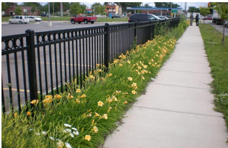
Example of Royal Oak Township's sidewalk infrastructure.
